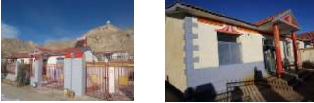
Figure 1: the test room-A single layer residential building with courtyard
