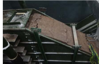
Figure 6: Overall destruction of landslide
