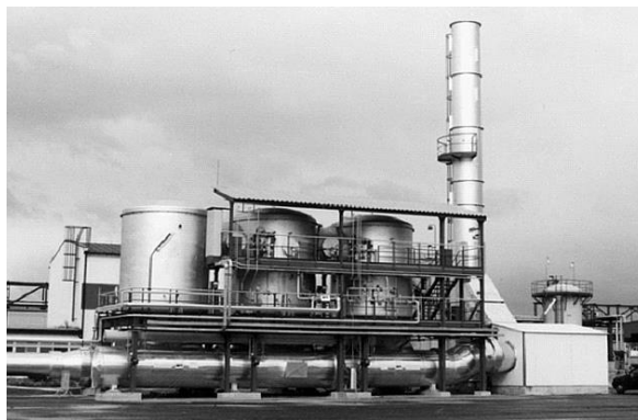
Figure 3: Photograph of the unit from Figure 2; regenerator consists of the two darker vessels left of the stack
