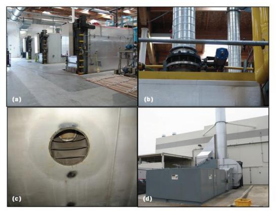
Figure 2: Sterilization chambers after facility reconstruction (a), <u>backvent</u> valve and duct (b), interior view of <u>backvent</u> (c) and catalytic oxidizer (d).
