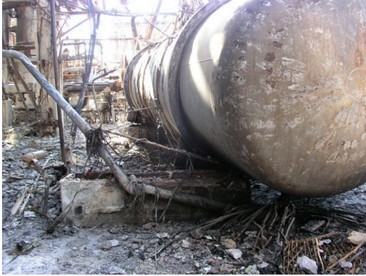
Figure 2 Tank Sliding in Long Dimension
