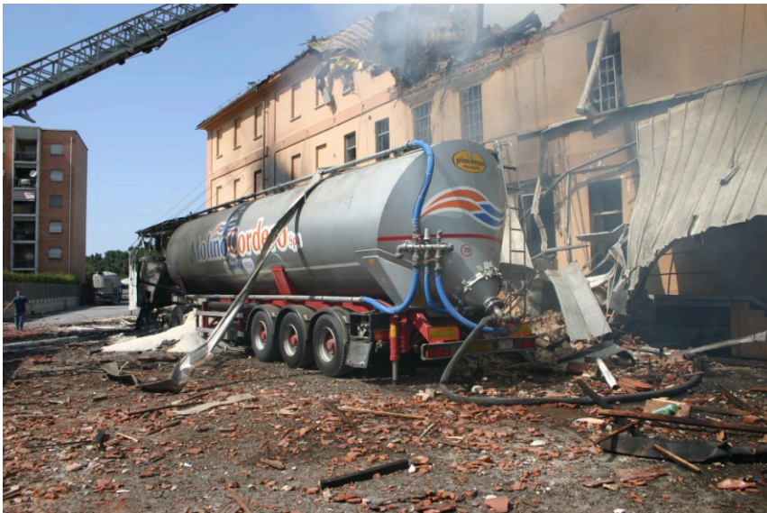
Figure 4 The tank after the accident
