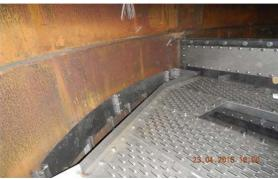
Figure 5a: Installation of the Dividing Wall in the FCC Naphtha Splitter at an Indian Refinery; Figure 5b: Dividing Wall Internals inside the Tower
