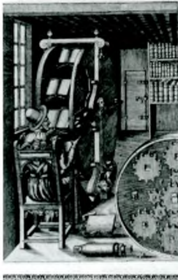
The reading wheel, from Agostino Ramelli's Le diverse et artificiose machine (Paris, 1588). Reproduced by permission of the Harry Ransom Humanities Research Center, University of Texas at Austin. 4
