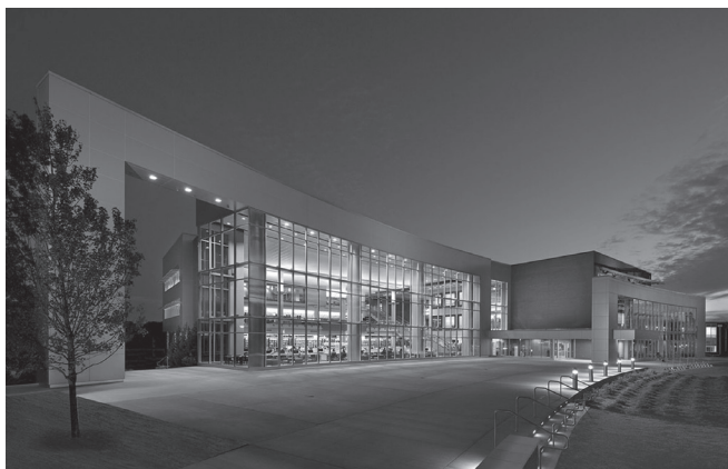
North façade and plaza at night at the Georgia Gwinnett College Library and Learning Center.
