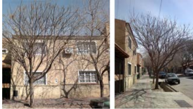
Figure 32. Case 4, Winter, (in the photograph, the shadow cast by bare branches on the North facade can be observed) and an appropriate value of SVF (tree top shadow partially occupies the surface of the street).
