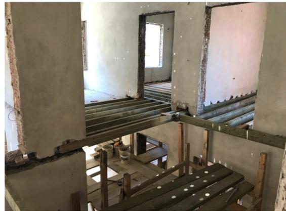
Fig. 12. Timber beams arranged between the walls
