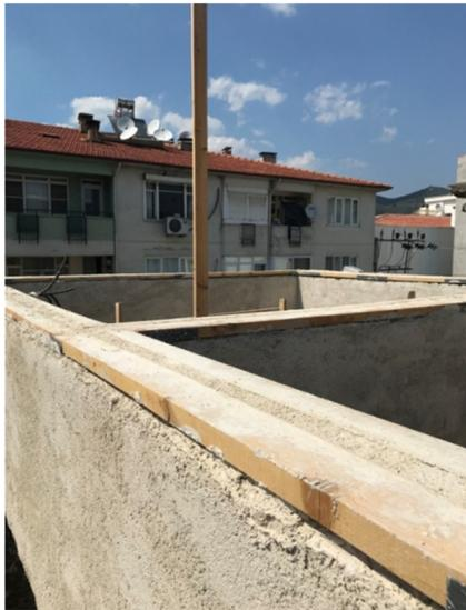
Fig. 10. The timber beams arranged on the top of the walls
