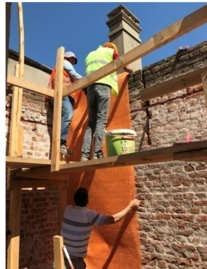
Fig. 8. The reinforcement of brick walls
