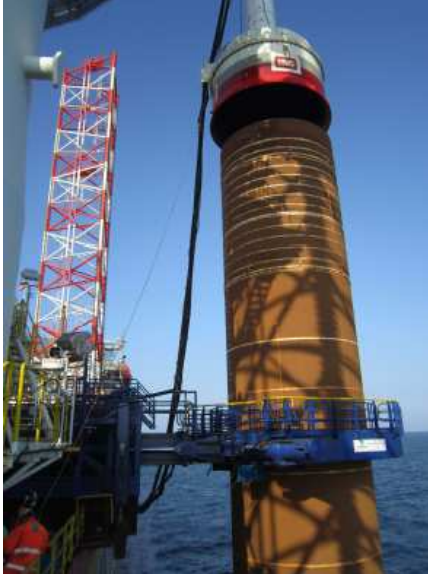
Figure 23. Pressing a pile by hydraulic pressure
