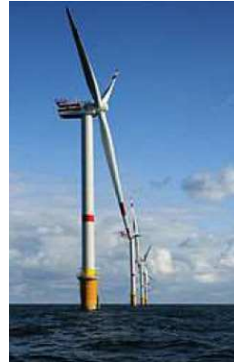
Fig.2. Wind turbine with horizontal axis of the Thornton Bank wind farm, Belgium
