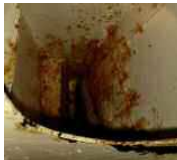
Fig.2. Example of a ship zone corroded under stress
