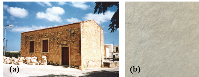
Figure 3: (a) Primary school at Scordilo village made of Alfas stone; (b) The compact texture of Alfas stone.
