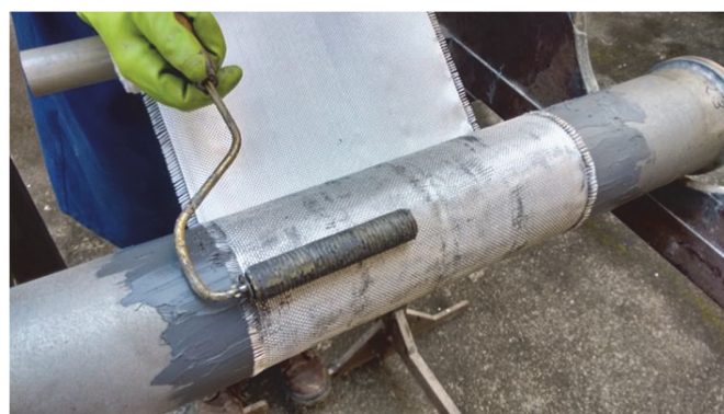
Figure 5: Pre-impregnated, bi-directional composite.
