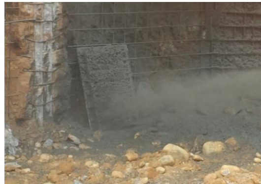
Figure 6: Shotcreting on wooden plates for sampling at tunnel site
