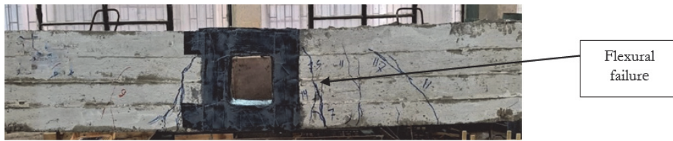
Figure 27: Failure mode for (B4M).
