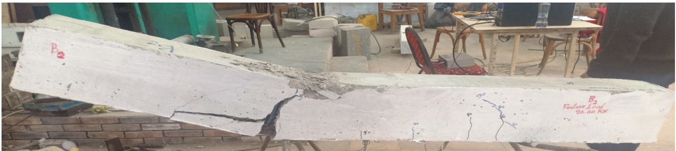
Figure 15: Concrete crack patterns at ECC beam (B 03) explain ECC groove rupture at tension surface.
