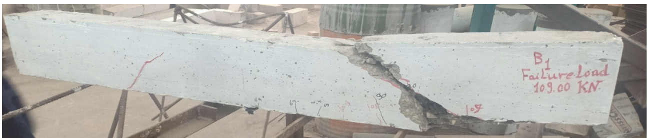
Figure 12: Concrete crack patterns at Epoxy beam (B 02) Explain the resulting cracks.
