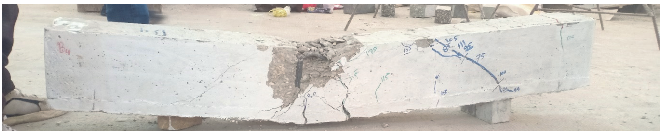
Figure 17: Concrete crack patterns at ECC beam (B 04) left side.
