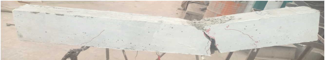
Figure 14: Concrete crack patterns at ECC beam (B 03).
