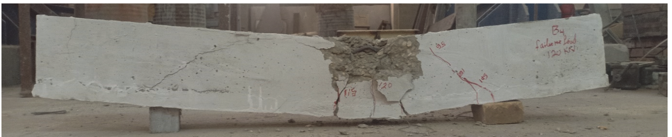
Figure 16: Concrete crack patterns at ECC beam (B 04) right side.
