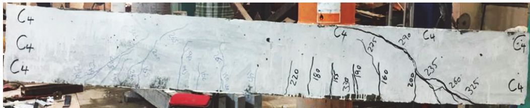
a) Control beam, C4.
