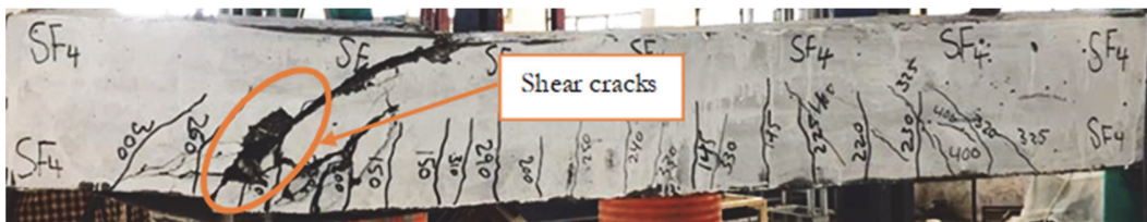
c) Steel fiber reinforced concrete technique, SF4.
