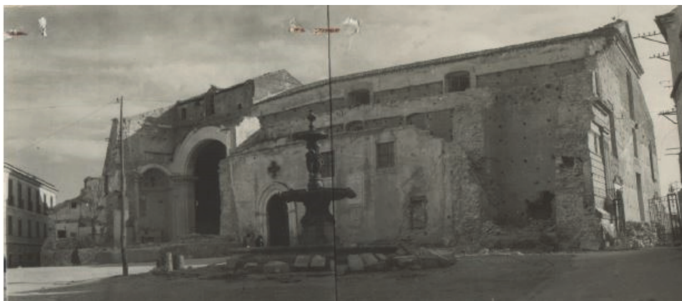
Figure 4: Left nave of Cathedral destroyed by World bombing. Calabria superintendency storage.
