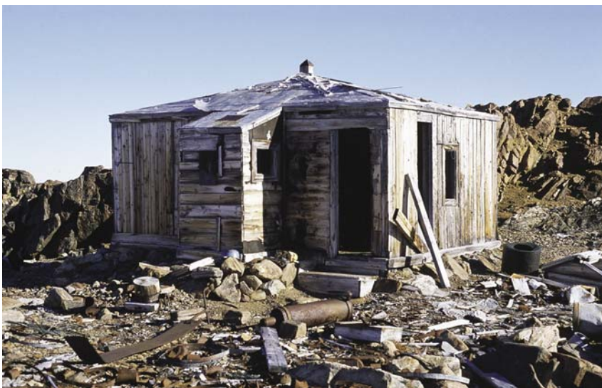
Fig. 26. Alabama, the hut on north-east Shannon built from timbers rescued from the ship ALABAMA that sank in its winter harbour nearby in March 1910. The hut is surrounded by a variety of debris from the ship, including a large rusty ice-saw in the left foreground.
