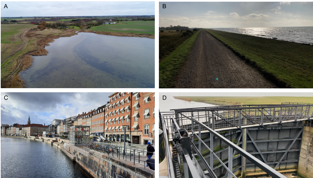
Fig. 10 Diversity of management options for extreme sea-level events. A: Coastal wetland in Roskilde Fjord, Sjælland. B: Earthen coastal protection dams near Rødby, Sjælland. C: Hardened shoreline at Copenhagen, Sjælland. D: High-water river lock on Ribe Å, Jylland.
