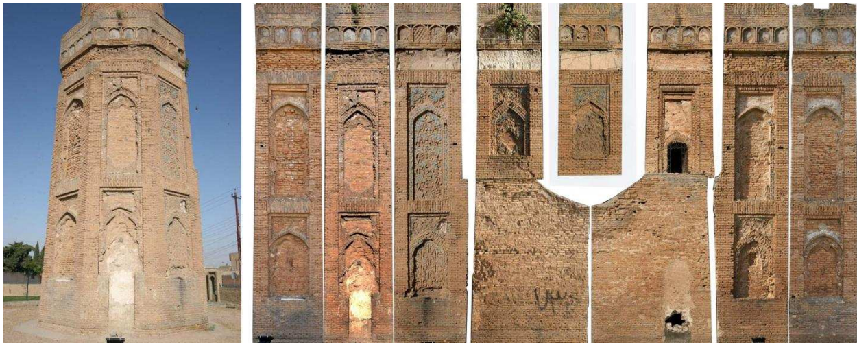
Figure 1: The Choli Minaret, Iraq, a: an image showing the lower part of the minaret, b: Rectified images of the different ornaments under investigation.
