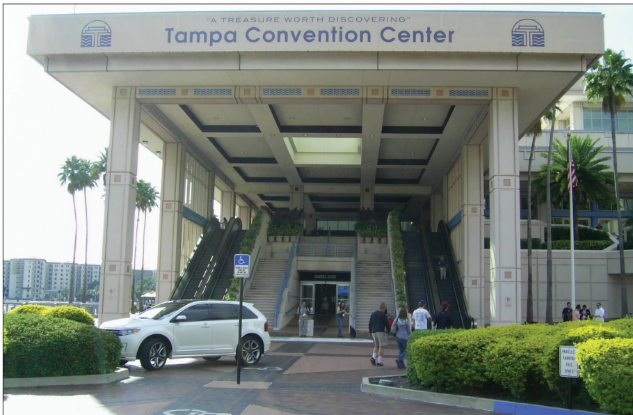
Tampa Convention Centre, channel entrance (Photo: SZABOLCS FABULA)
