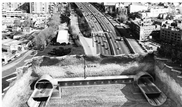
Figure 2. Southern by-pass cross-section (ACCIONA-Infraestructuras).
