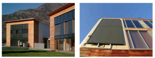
FIG. 1 Left. Glazed flat plate collector integrated into a modular façade system (Winkler Solar, n.d.), Right. Prototype of unglazed collector integrated into a metal cladding panel (Elguezabal, Garay & Martin, 2017).
