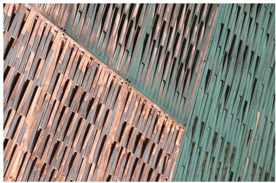
FIG. 3 Sense Envelope III. Copper and polypropylene are forming a thermally active composite. Design/fabrication by Isak Worre Foged and Anke Pasold. Photograph by: Isak Worre Foged.
