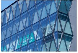
FIG. 2 J6 Front in Tokyo Omotesando (by architect Matsuda Hirata Design Inc., 2008) features a diagrid of structural supporting elements with a diagonal grid of façade elements.
