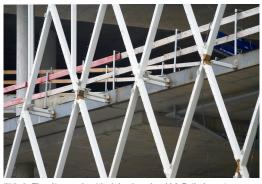
FIG. 3 The diagonal grid of the façade of MyZeil shopping centre in Frankfurt am Main (by architect M. Fuksas, 2009). The façade smoothly transforms into the triangulated geometry of the free-form roof. The figure shows the substructure of the façade grid attached to the floor slabs before the façade profiles were mounted.
