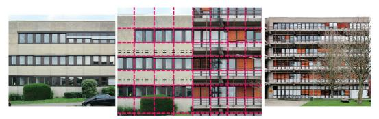
FIG. 1 Regular horizontal and vertical grids of office buildings
