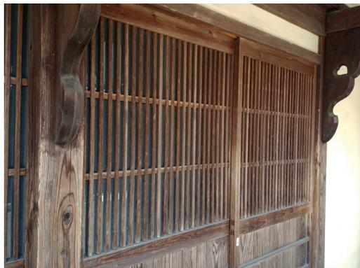
FIG. 3 *Koshi* placement close to the exterior window surface in a house, in Uchiko, Ehime
