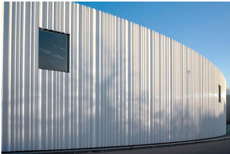
Fig. 4. Completed façade section (Image: Michel).
