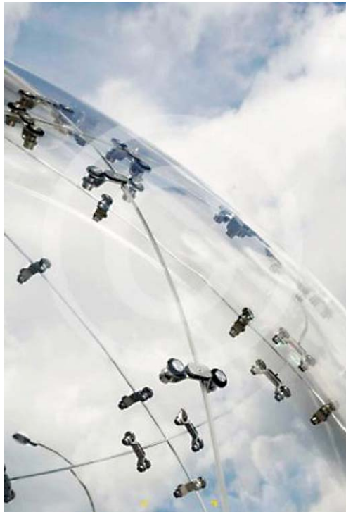
Fig. 1. Acrylic glass as a substitute for glass: joints with point fixtures on the acrylic glass shell of the BMW hourglass (Photo: Photodesigner).
