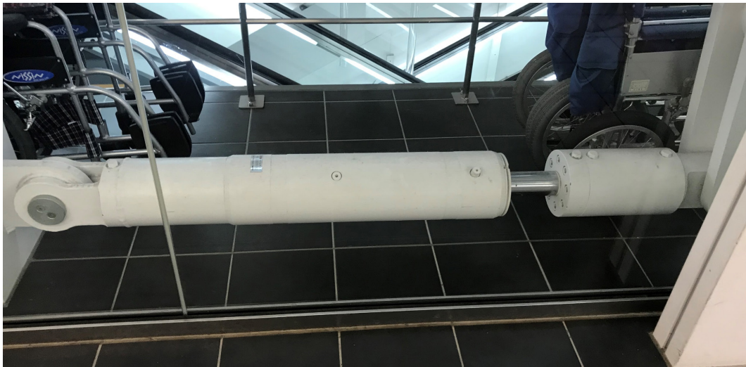
FIG. 3 A viscous fluid (VF) damper manufactured by KYB Corporation, Japan
