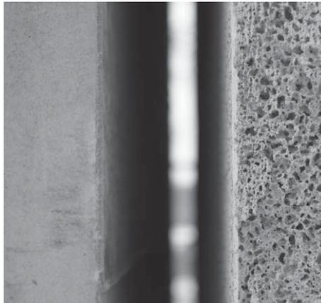
**Fig. 14.** Facade panels made of UHPC (left), insulating layer of mineralized foam (right).
