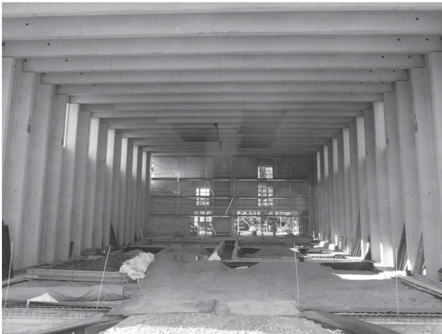
**Fig. 10.** Interior view of the rib structure of the industrial hall.
