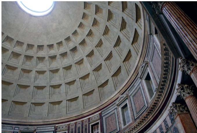
Fig. 9. Pantheon Rome, View of the oculus. One of the first 'concrete (opus caementitium)' buildings.
