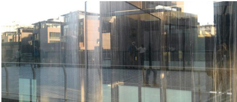
**Fig. 1.** Example of significant water stains on a facade, caused by lack of maintenance action.
