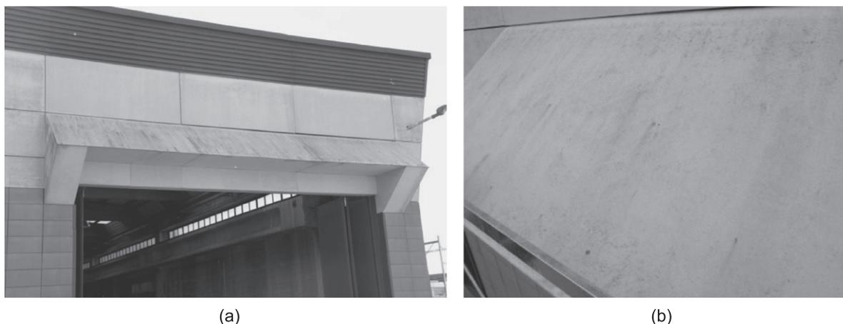
**Fig. 11a–b.** Heavy soiling deposits on the protection canopy (silica-calcium cladding).
