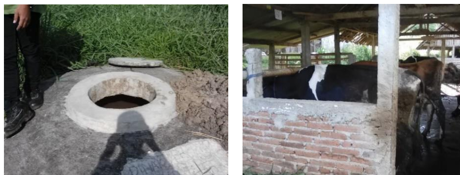
Fig 12. Tank Installation of Biogas & Communal Sheds
