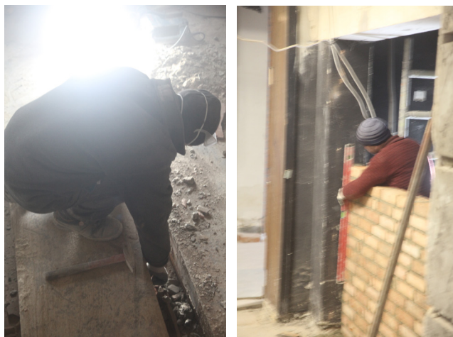
Figures 7 and 8 From the series The Construction Site of Remembrance (2018–21).
