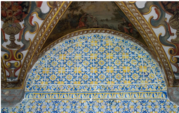
FIGURE 7 | Arches of the vaults in the lower-choir.
