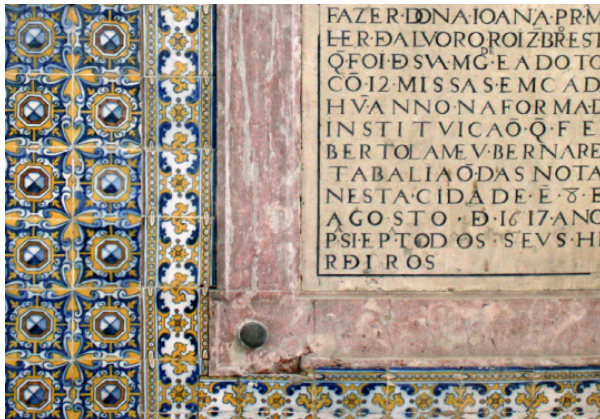
FIGURE 4 | Chapel of Dona Joana Pereira. Detail of the frames used as a bar overlaid tile strands) (see Figure 4).
