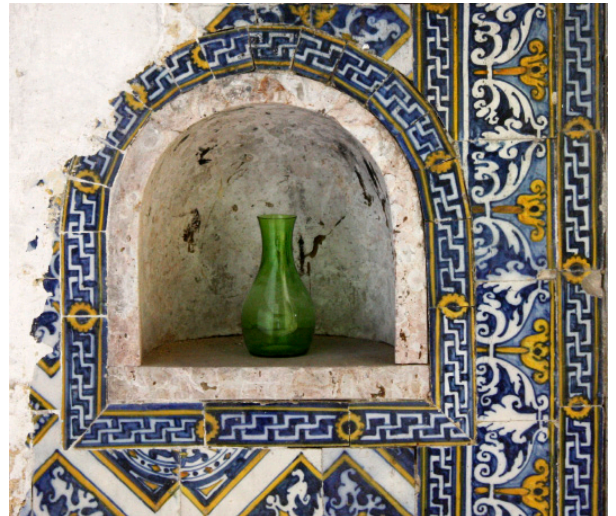
FIGURE 6 | Chapel of the Brotherhood of Glorioso Santo António. Detail of the niche with a frieze.
