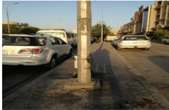
Figure 14: Obstacles in the pedestrian paths that left no space for walking (Ref: the Researcher)
