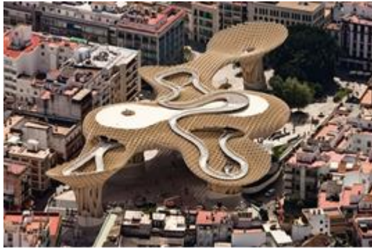
Figure 4: Shading with wood structure (Jurgen- Mayer from Seville, Spain)
