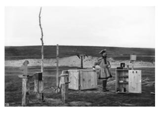
**Fig. 3** Sophus Tromholt's auroral observatory in Kautokeino 1882–83. In the middle of the picture you can see the Mohn theodolite, which was used in triangulating the position of the aurora. (Photo by Sophus Tromholt, courtesy of the University of Bergen Library.)
