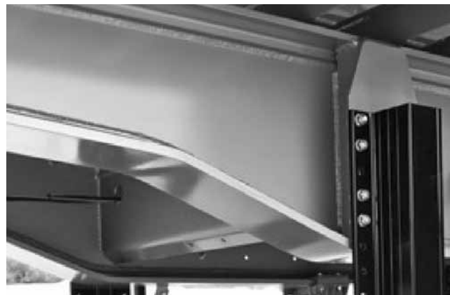
Rys. 11. Spoina gotowa do odbioru Fig. 11. A view of a weld on a completed vehicle
