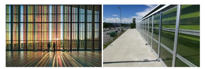
**Figure 6.** Examples for DSSC-based photovoltaic glazing. Left: DSSC panels produced by the company Solaronix (www.solaronix.ch) mounted at the façade of the Swiss High-Tech Convention Centre in Lausanne, Switzerland. Right: The first energy-producing noise-barrier based on the DSSC panels developed by the Swiss company H.Glass is installed on the highway between Bern and Zurich in Switzerland.
