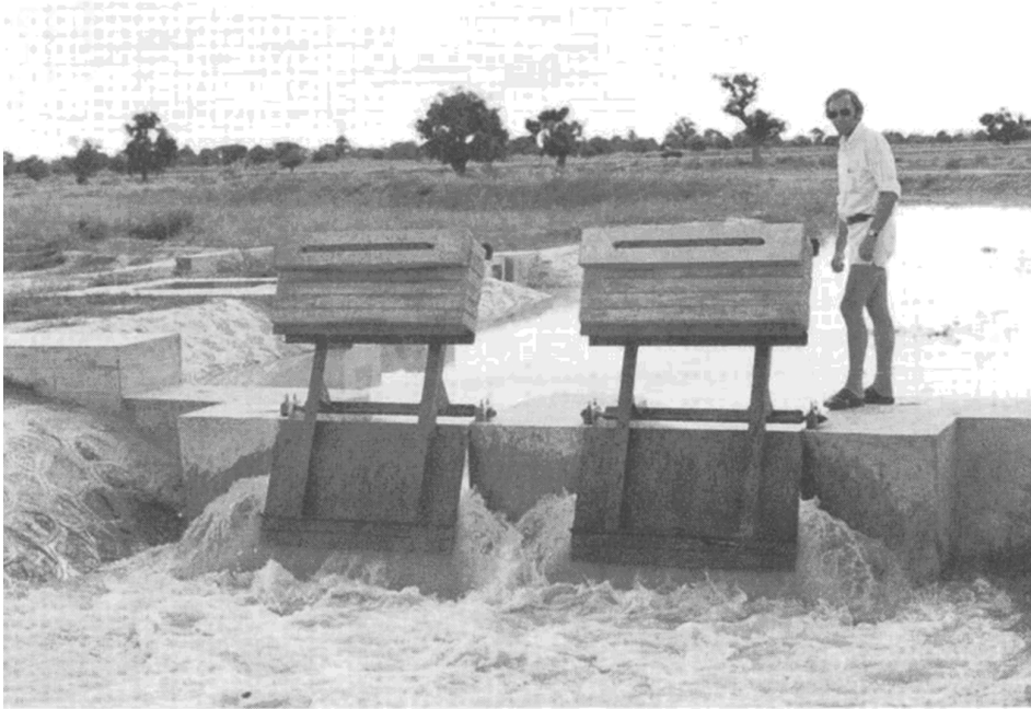
Figure 1. Begemann Gates in the Kano River Project. Source: Private archives of R. Brouwer
