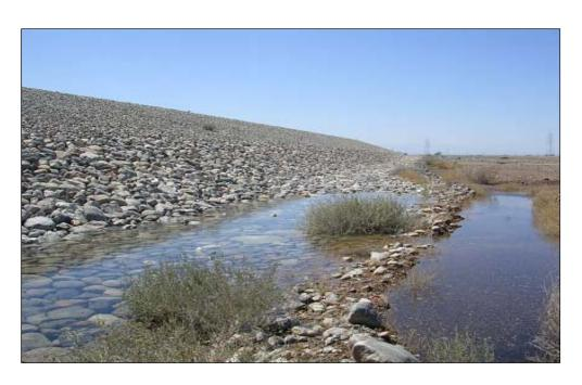
Figure 3. Seepage from the dam.
