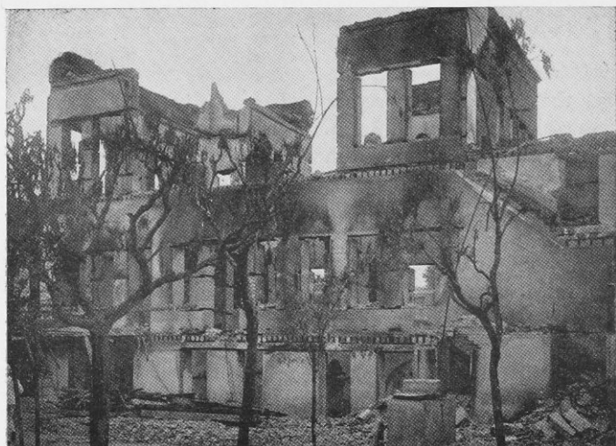
THE BOARDING-SCHOOL OF THE SISTERS OF ST. JOSEPH AFTER THE FIRE.
