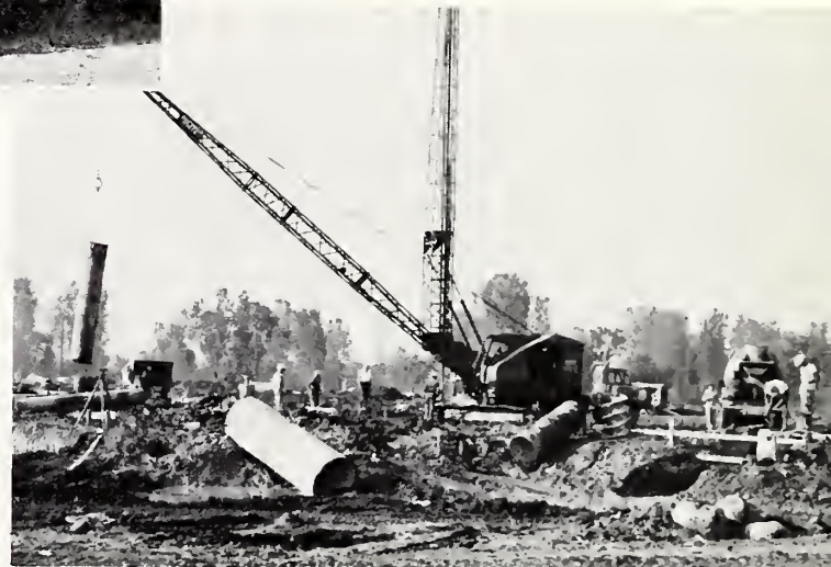
First stage of construction was driving of 404 concrete caissons for foundation.
