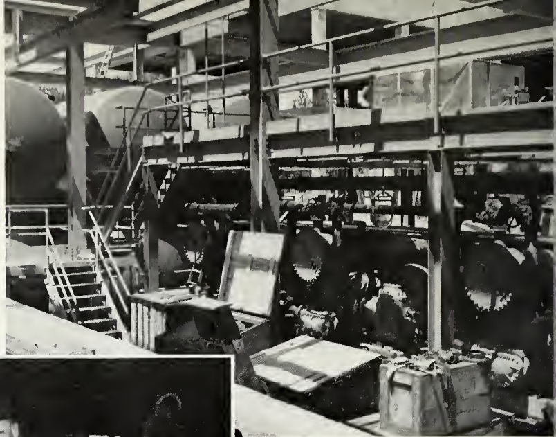
Early stages of the construction of heat pump.
