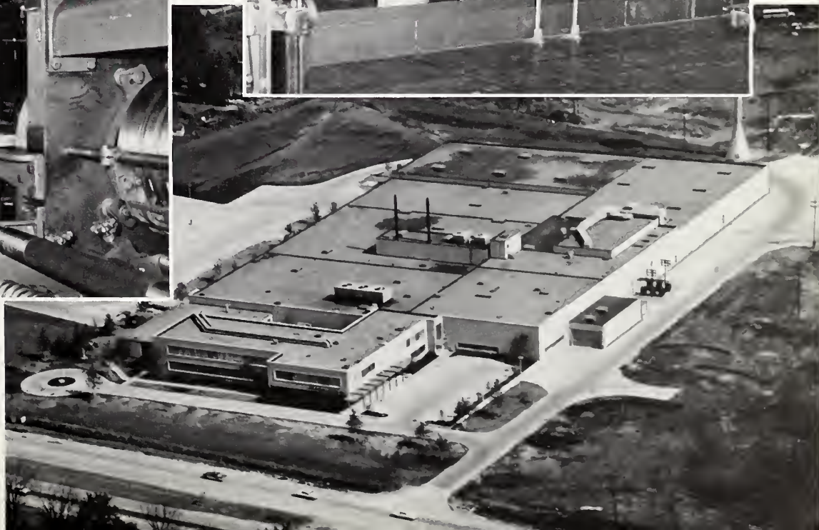
As building appeared in final stages of construction.
