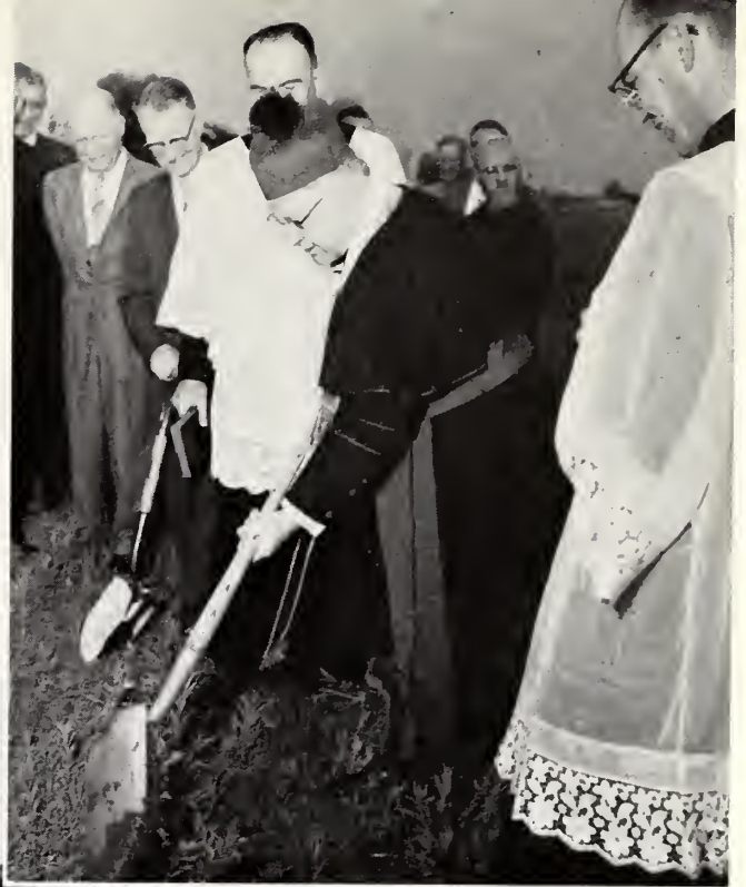
... with ground-breaking ceremonies at which Bishop Pursley officiated on May 25, 1959.
