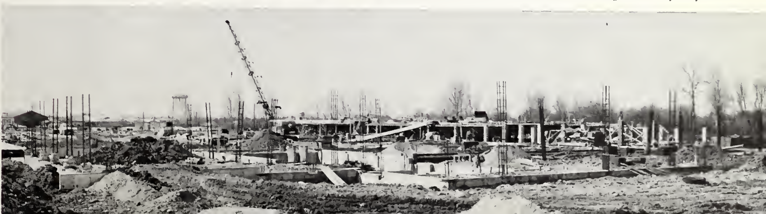
As building began to take shape in early days.
