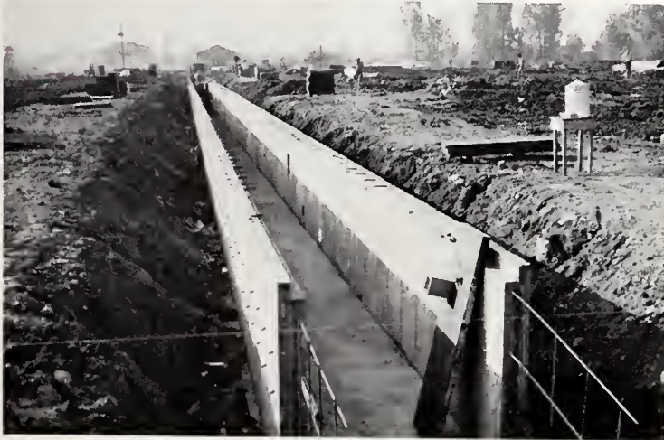
Tie-in trench for underground utilities.
